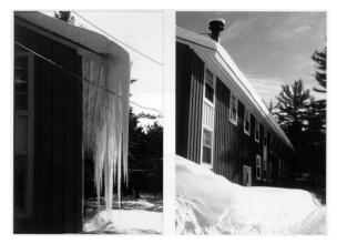
*Figure 1* Two identically constructed roofs photographed at the same time. The one on the right, with no icings, was unheated.
